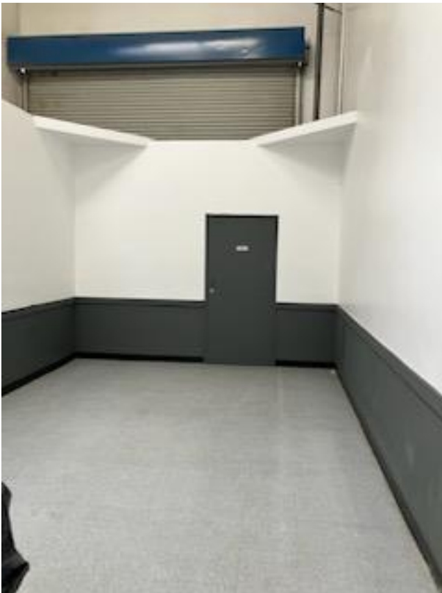
Power Play party rooms completed 2/23/24
